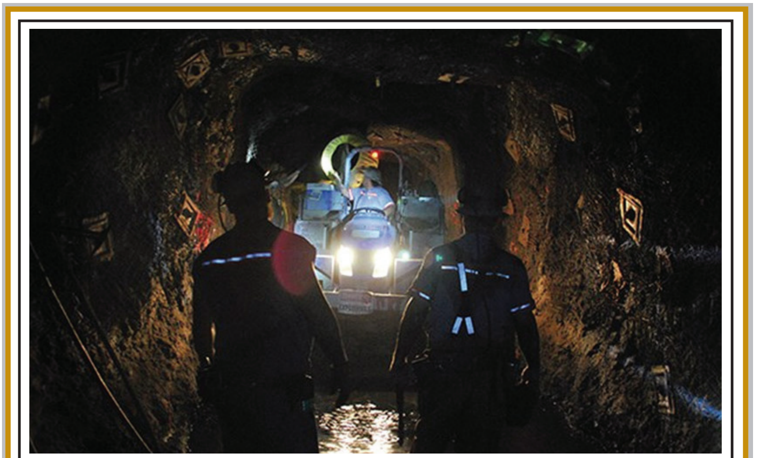
Turquoise Ridge has the highest average reserve grade in the Company's operating portfolio. Construction during the first quarter centered on well drilling activities, electrical distribution, and mine site utility construction and activation.
