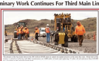
The project is the key to the new $2.5 billion BNSF plan to expand its main line in the state. About 10% of the project is completed and construction on 1,000 miles of track and replacing 17 miles of rail will start in 2020.
